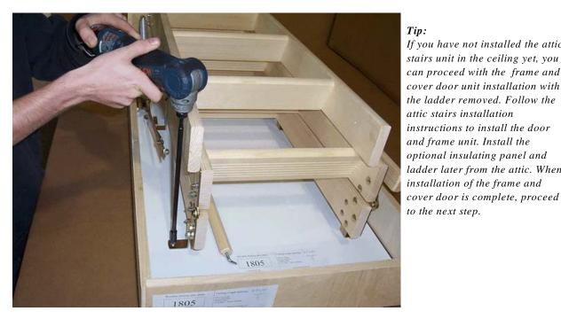
If you have not installed the attic stairs unit in the ceiling yet, you can proceed with the frame and cover door unit installation with the ladder removed. Follow the attic stairs installation instructions to install the door and frame unit. Install the optional insulating panel and ladder later from the attic. When
